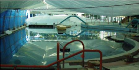
Figure 7.12 – Pool tank is filled with water during the flood test stage. Upon successful flood testing, the pool will be drained, dried and ready to be tiled (as a side note, notice the tenting that is protecting the water feature from the elements during the installation and curing process).
