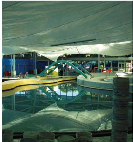
**Case Study 10** – The swimming pool is now in the flood test stage. The waterproofing membrane must be allowed to reach its full cure prior to flood testing. Full cure will vary by manufacturer and product type. The pool is filled at a rate of 1" (25 mm) per hour. Generally the water level will be continually monitored during the length of the flood test (typically 24 - 72 hours) to determine a vessel's 'water-tightness'. The water is then drained at a rate of 1" (25 mm) per hour.
