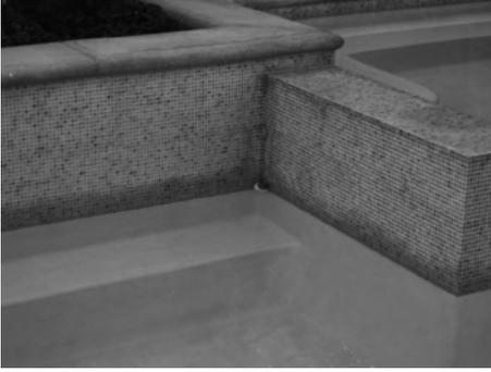
Figure 12.14 – Notice the difference in color between the tile and grout above the water line and below the water line. This condition is typical because cement-based grout absorbs water and creates the darker look at the water line. Expectations should be managed accordingly.
