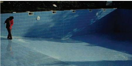
Figure 7.19 – View of completed swimming pool. Note the movement joint at the changes of plane on the floor of the pool and the other field movement joints on the walls and floors.
