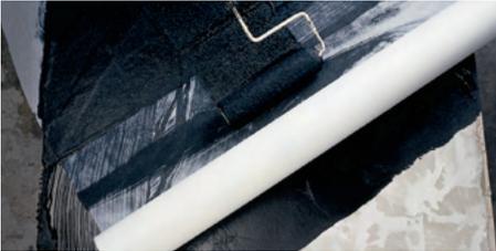
Figure 7.8 — Liquid applied membrane applied to concrete substrate.
