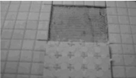
Figure 12.11 – Large PVC dots on rear/edge mounted porcelain mosaic tiles can lead to bonding issues as is evidenced from these photos. Latex fortified portland cement based thin set mortars may have a difficult time achieving a sufficient bond to the PVC rubber. The PVC dots are covering 50 – 60% of the tile back. An epoxy adhesive may be required to install tile mounted in this fashion in wet area and continuous submersion applications.
