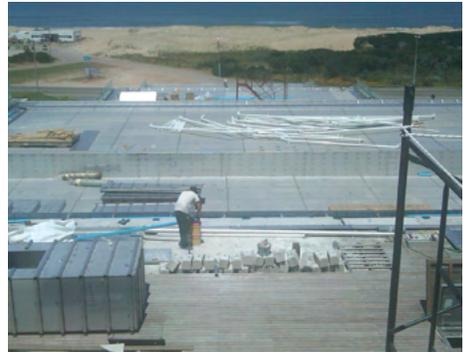
Figure 3.2 — steel pool shell being installed in Uruguay.
