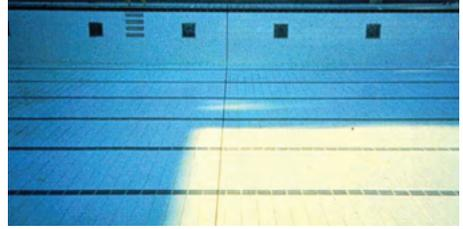
Figure 7.20 – View of completed swimming pool. Note the movement joint running continuously through the width of the swimming pool both at the walls and floors. A properly placed water stop in the concrete shell is a critical design element to ensure system functionality.
