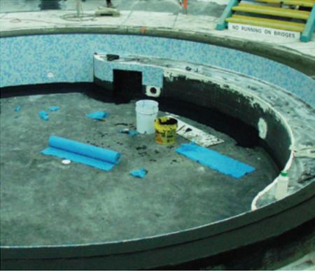
**Case Study 11** – The tile installation can now begin. Generally, work begins on the vertical areas first. A high strength liquid latex fortified thin set mortar (e.g. 257 Titanium) suitable for submerged applications is used. Care is required when working over the waterproofing membrane.
