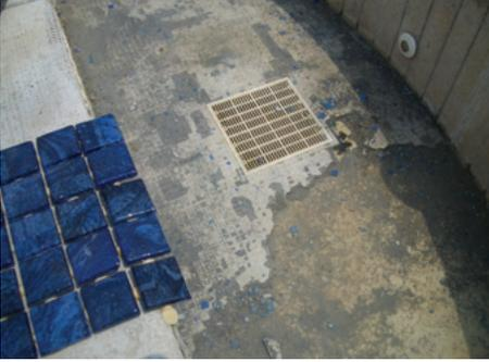
Figure 12.6 – The increased use of prefabricated tubs (e.g. fiberglass or stainless steel) requires the use of a 100% solids epoxy adhesive (e.g. LATAPOXY 300 Adhesive). In this instance, a typical latex fortified portland cement based thin set mortar was used over a fiberglass tub that resulted in bond failure.
