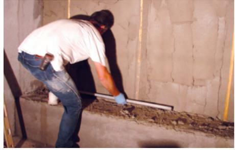
Figure 7.2 — Latex fortified render is being applied to wall surface. Notice the lath strips that are set into the mortar. The lath strips are leveled and plumbed to establish the correct wall render depth. Once the render achieves a sufficient cure, the lath strips are carefully removed and the cavities are filled with mortar.
