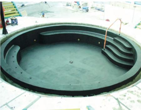
**Case Study 8** – The waterproofing installation is complete. The waterproofing membrane must be allowed to fully cure prior to the flood test. Full cure rates will vary by product type. Consult with the waterproofing manufacturer for full details.
