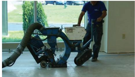
Figure 6.6 – Shot-blasting is ideal for areas outside of pool tanks and water features and for areas where access by the equipment is not an issue.
