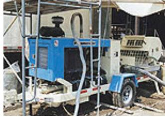
Figure 6.18 – Mortar is mixed and pumped to area in a combination mortar mixer/pump combination.
