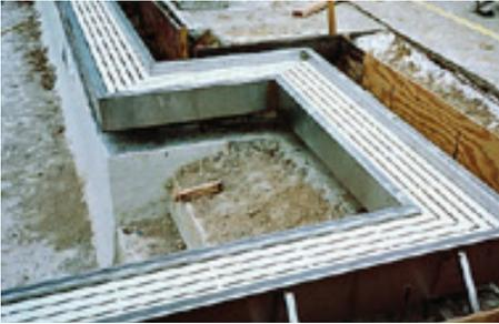
Figure 7.5 — Stainless Steel Pool Gutter Assembly. Tile or Stone is brought up to the gutter assembly in the tank and on the deck (Photo courtesy of Barrier Lining, Inc.)
