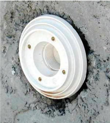
Figure 4.7 – Return port in a concrete shell pool<sup>8</sup>.
