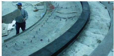
Figure 7.4 — Mechanic is using a wooden template to shape and screed the swale in the water feature tank.
