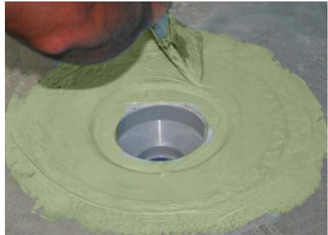
Figure 12.4 – The liquid applied waterproofing membrane must be flashed into a two part clamping style drain to create a watertight seal.
