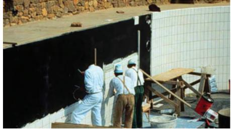
Figure 7.13 — Installation of mosaic tile with liquid latex fortified portland cement thin-set mortar.
