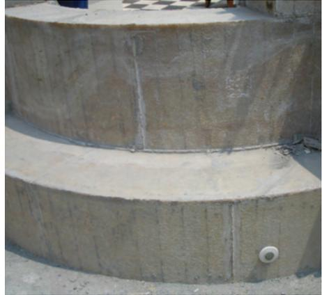
Figure 3.4 – A fiberglass pool shell waiting installation of tile.
