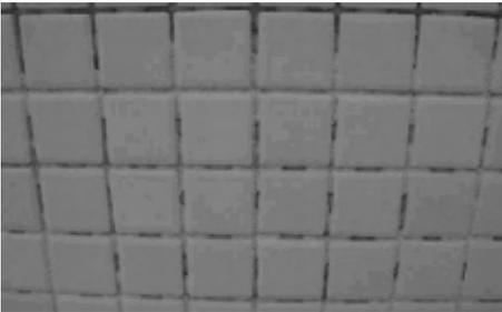
Figure 12.15 – Erosion of grout joints is the diagnosis on this application. Possible causes are as follows:
