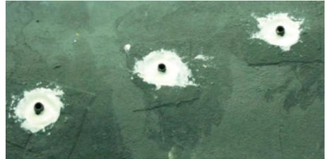
Figure 7.7 — Epoxy waterproofing membrane is applied at the pipe penetrations over the cured liquid applied waterproofing membrane to ensure a complete seal at the penetrations.
