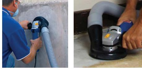
Figure 6.5 – Saw Tec® Dustless Grinding. This method is ideal for spot preparation and solves localized problems.
