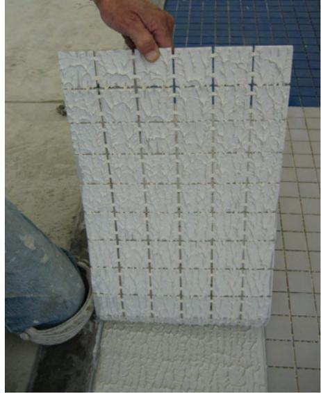
Figure 12.9 – It is good practice to periodically lift / remove freshly installed tiles or stones to verify that a minimum 95% continuous adhesive mortar is achieved. If the desired coverage is not achieved, use a larger trowel to dispense adequate adhesive mortar and beat-in the tiles correctly to achieve the desired results.
