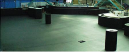
Figure 7.11 – Waterproofed pool tank is curing and awaiting a flood test. Curing term of waterproofing membranes can vary by manufacturer. Consult with waterproofing manufacturer for detailed information on cure rates and flood testing processes.
