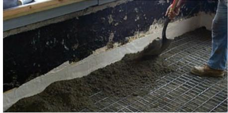
Figure 8.1 – Example of a non-bonded, wire reinforced mortar bed. Wire mesh is placed in the middle of the mortar bed and lapped together to ensure continuity.
