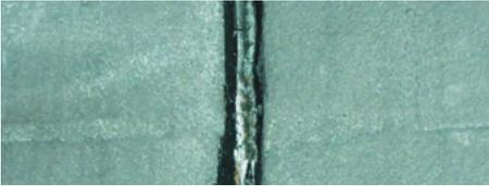
Figure 7.17 – Waterproofing reinforcing fabric is then folded and placed into the movement joint and folded onto the concrete/mortar bed. Additional waterproofing liquid is applied over the treatment. A third coat of liquid is then applied to seal off the entire treatment.
