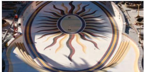
Figure 7.15 — Mosaic tiled stainless steel pool tank. Only an epoxy adhesive can be used to install tile directly to steel tanks. (Photo courtesy of Bradford Products, LLC.)
