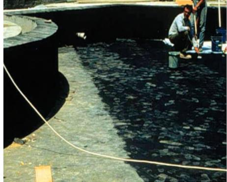
Figure 12.3 – Once the waterproofing membrane is applied, it should be protected from traffic and work from other trades.
