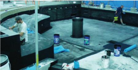
Figure 7.9 — Full scale view of liquid applied waterproofing membrane on a large scale pool project.
