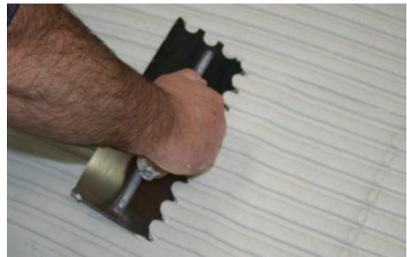
Figure 7.1 — Trowel applied large, heavy tile mortar with a 3/4" (19 mm) loop notch trowel.
