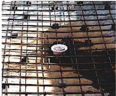
Figure 4.5 – Typical drain position and steel reinforcement prior to gunite application of concrete.
