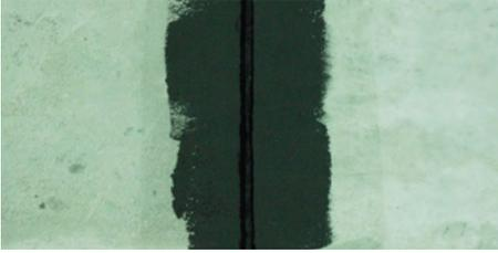
Figure 7.16 – Waterproofing liquid is applied onto the sides and into the expansion joints.
