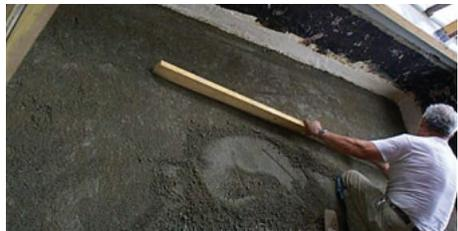
Figure 8.2 – Tile mechanic screeding an unbonded mortar bed.
