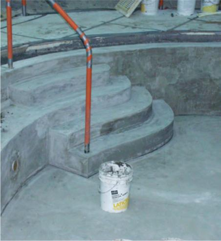
**Case Study 3** – The use of a LATICRETE® liquid latex fortified portland cement based leveling mortar is used to correct any irregularities in the concrete shell. Proper surface preparation will result in an aesthetically pleasing tile or stone finish.
