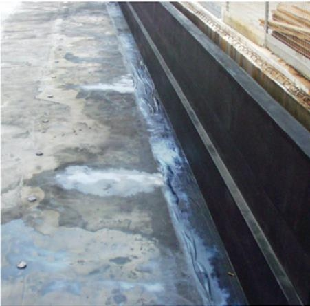
Figure 12.2 – Effects of exposure to rain prior to the waterproofing membrane reaching its full cure. This damaged waterproofing membrane will need to be removed, reinstalled, protected and allowed to reach its full cure.
