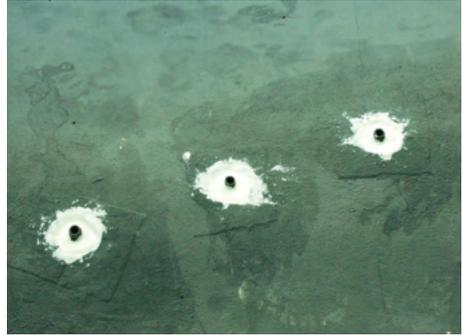
**Case Study 9** – The penetrations are sealed with a suitable flexible sealant. Generally, 100% silicone sealant (e.g. Latasil™ with 9118 Primer) or urethane sealant with non-solvent based primers can be used. All precautions to create a complete watertight tank must be taken to ensure a successful flood test.
