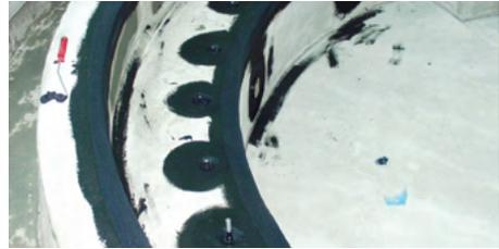
Figure 7.10 — Detail treatment of the pipe penetrations in this pool application. Liquid applied waterproofing membrane is double applied at the penetrations to ensure adequate reinforcement and protection. This pool is now ready for the full waterproofing treatment.
