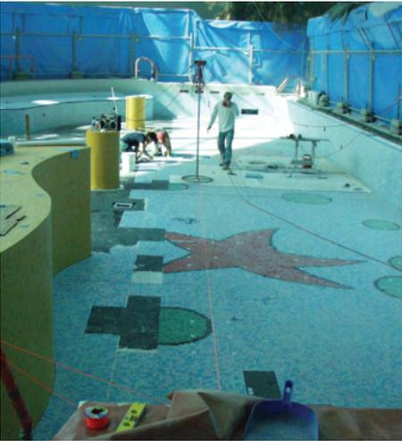
**Case Study 12** – The installation of the tile in the horizontal areas is now complete. Once the tiles are installed and grouted; the installation must cure for a full 14 days after the final grouting period at 70°F (21°C) if a latex fortified portland cement based grout (e.g. PERMACOLOR™ Select Grout) is used or 10 days if an epoxy based grout (e.g. SPECTRALOCK® PRO Premium Grout\*) is used.
