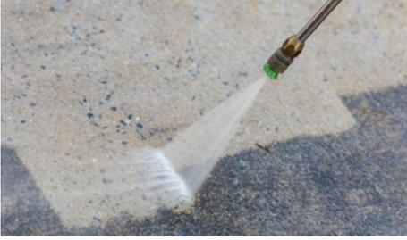
Figure 6.7 — High pressure water wash (water-blasting) may remove the required amount of contaminated concrete.
