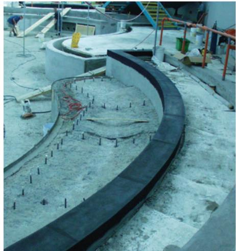
**Case Study 2** – Mechanic is using a wooden template to shape and screed the swale in the water feature tank. Latex fortified portland cement mortars and renders are used for this purpose.
