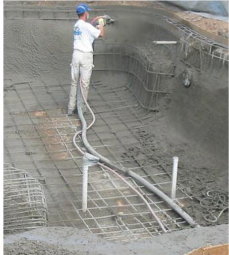
Figure 3.1 — Gunite being sprayed and finished in a residential pool.
