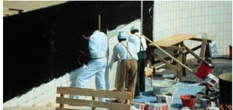
Figure 7.14 — Installation of glazed porcelain tile with liquid latex fortified portland cement thin-set mortar over a liquid applied waterproofing membrane.
