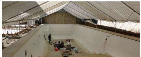
Figure 6.3 — Outdoor pool work done with tenting regulate temperature.
