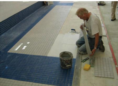
Figure 12.8 – Only enough latex fortified portland cement thin set mortar is spread to allow the installation of the porcelain mosaics within the mortar's typical open time – generally 15 minutes at 70°F (21°C).
