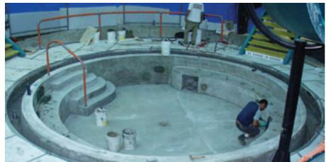
Figure 7.3 — Tile mechanics float and shape pool utilizing templates, floats and screeds to achieve the desired form and height of the renders and mortar beds.
