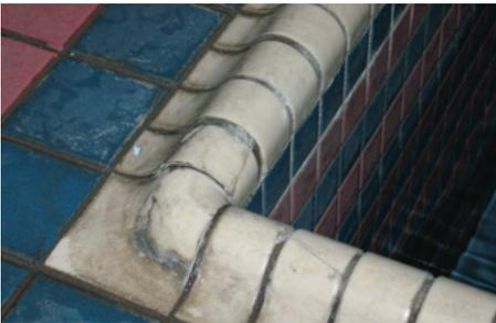
Figure 7.6 — Uniquely shaped pool/deck rim which required careful forming of the render in order to place the finished tile.
