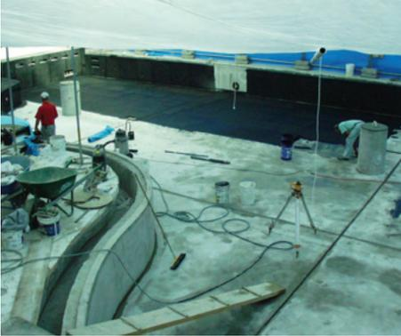
Figure 12.1 – Exterior applications must be protected from the elements during the installation and installation materials cure periods. A temporary tent was erected over this swimming pool to protect the application from direct sunlight, wind and rain.
