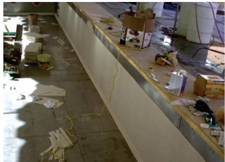
Figure 12.5 – Steel pool tank. Porcelain mosaic tiles are installed with a 100% solids epoxy thin set mortar adhesive (e.g. LATIPOXY® 300 Epoxy Adhesive) to achieve a suitable bond to the steel tank assembly.
