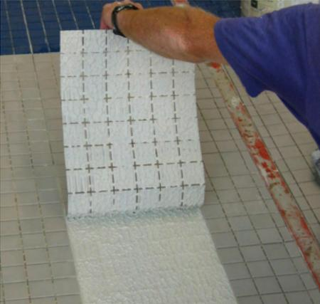
Figure 12.7 – Porcelain mosaic tiles installed on pool deck. Notice the ribbons of latex fortified thin set mortar combed in one direction to maximize coverage.
