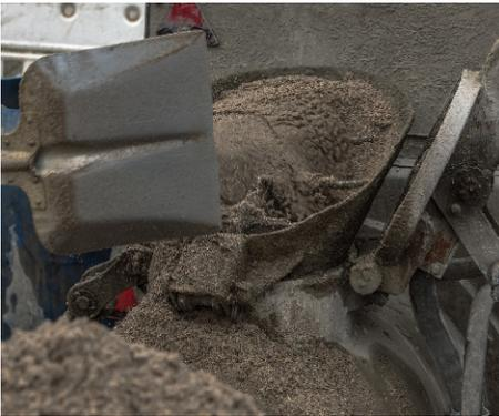
Figure 8.16a — Vibrated floor process — Mortar is mixed and pumped to area in a combination mortar mixer/pump combination.
