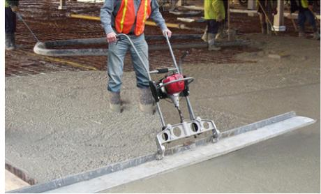
Figure 8.16c — Vibrated floor process — mortar is screeded with a vibrating screed to the desired height and pitched.
