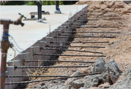
Figure 2.25 — Showing placement of shear connections and edge detail.
