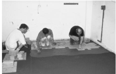
Figure 8.16e — Vibrated floor process — epoxy slurry bond coat is troweled onto fresh screed. Porcelain pavers are installed into the fresh epoxy slurry bond coat.
