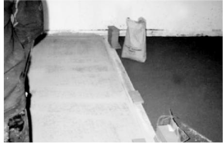
Figure 8.16d — Vibrated floor process — floor is squared and prepared to receive quarry tile floor.
