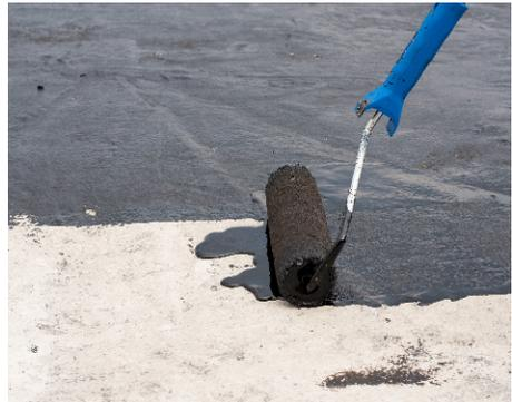
Figure 6.1 – Liquid applied membrane applied to concrete substrate.
