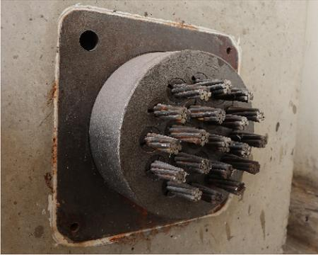
Fig. 2.21 — Post Tensioned Concrete Slab — Photo Courtesy of Suncoast Post Tensioning Company.
