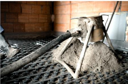
Figure 8.16b — Vibrated floor process — screed mortar is discharged onto floor area from the mortar pump.
