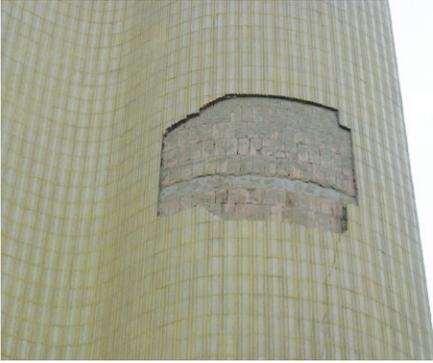
Figure 5.2 – Result of improper tile selection for the application. The use of a semi-vitreous tile – 7% in absorption did not stand up to the demands of this installation.
