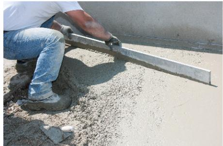
Figure 7.7 – Tile mechanic screeding a mortar bed.
