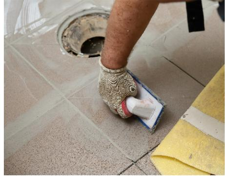
Figure 7.12 – Spreading of industrial epoxy grout.
