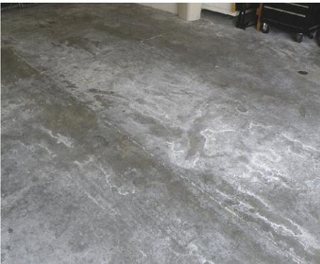
Figure 2.19 — Presence of Efflorescence on surface of concrete slab. Moisture migration through the slab can carry destructive salts to the surface of the concrete slab.
