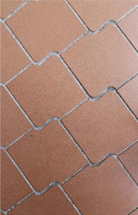
Figure 5.5 – Quarry Tile Floor – Photo courtesy of The Flooring Factory.
