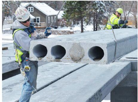
Figure 2.24 — Pre-Cast Concrete Planks. Planks rest and are supported by a flange attached to the steel girders. The planks are hoisted into place by a crane and mortared to the beams and to each other. Photo courtesy of Country Materials Corporation.<sup>16</sup>
