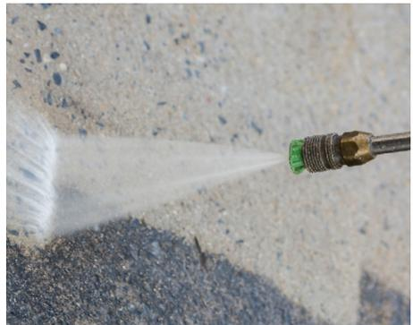
Figure 3.2 – High Pressure Water Washing.
