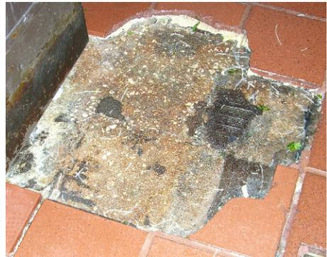
Figure 7.9 – Effects of inappropriate grout used on an industrial application. Notice not only the erosion of the grout joints, but also the adhesive mortar under the tile. In most industrial floor applications, the use of an epoxy-based adhesive and an industrial epoxy grout are required in order to ensure long-term performance.
