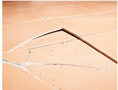
Figure 2.4 — Result of stresses induced by concrete shrinkage and lack of movement joint control. As the concrete shrinks, expansion joints are required to relieve the stress. When expansion joints are omitted or are not sufficient, “tenting” of the tiles can occur, creating bond failure and cracking.
