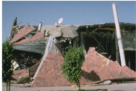
Figure 7.2 — High adhesive shear and tensile strength to resist seismic movement. Photograph of the Bullocks building after the Northridge California earthquake in 1994. Tiles remain adhered after severe shear stress from seismic activity and structural failure.
