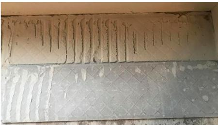
Figure 8.6 – Example of incomplete bedding due to lack of sufficient mortar and/or incorrect trowel size selection and beat-in.
