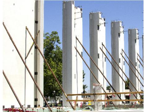
Figure 3.1 – Tilt-Up Concrete Panels erected into place.
