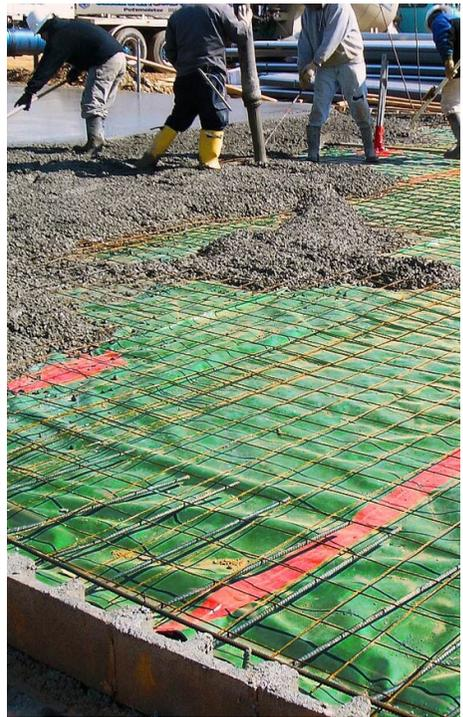
Figure 2.13 – Placement of vapor retarder over blatter layer / directly under the concrete pour.
